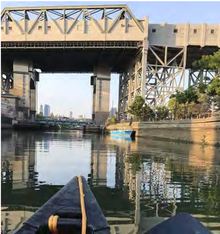
6/15/17 Photo of Culver Viaduct, Gowanus Canal
