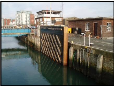
Miter gate in open position.
