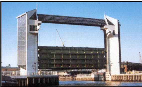
Barrier lifting gate in semi-lowered position above water.
