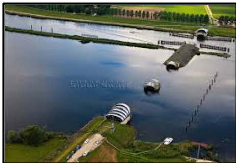
Rubber dams in deflated open position.
