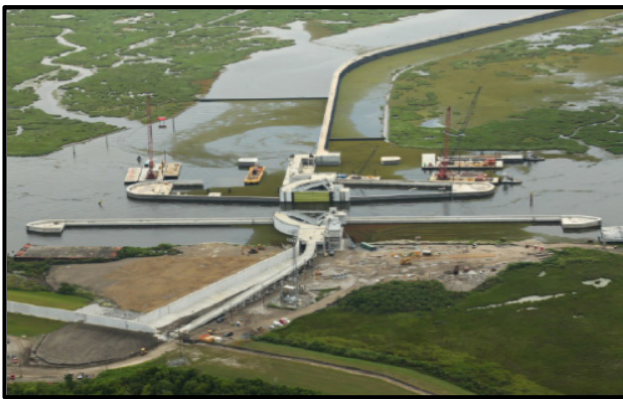
Overall aerial view of barrier. Source: USACE, 2012
