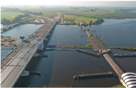
Overall aerial view of barrier.
