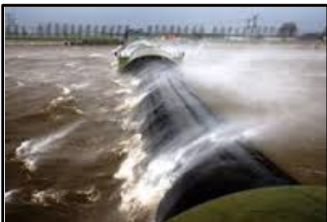
Rubber dams in inflated closed position.
