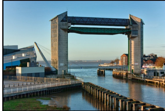
Hull Barrier, UK – Lifting gate in normal open position rotated 90 degrees to maximize navigation clearance
