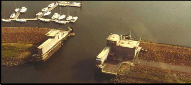
Aerial view of barrier with gate in open position lying flat on channel bed. Source: USACE, 2008
